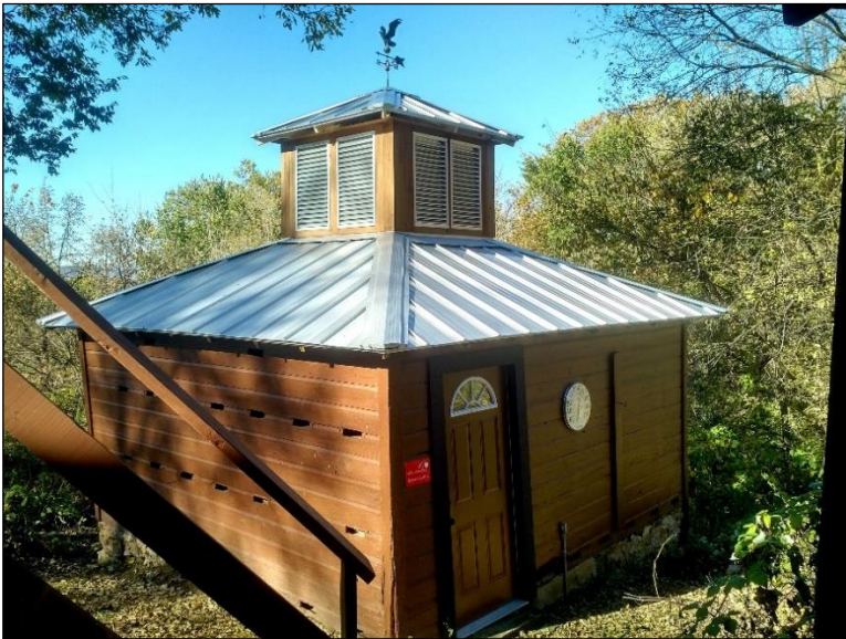
Thrive! Center Beehouse, Renovated/Restored, 1885 Era
